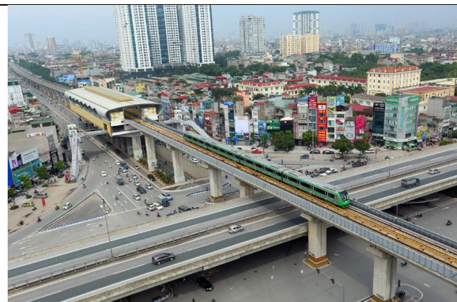
Fig 40: Hanoi metro line 1 is nearing completion
